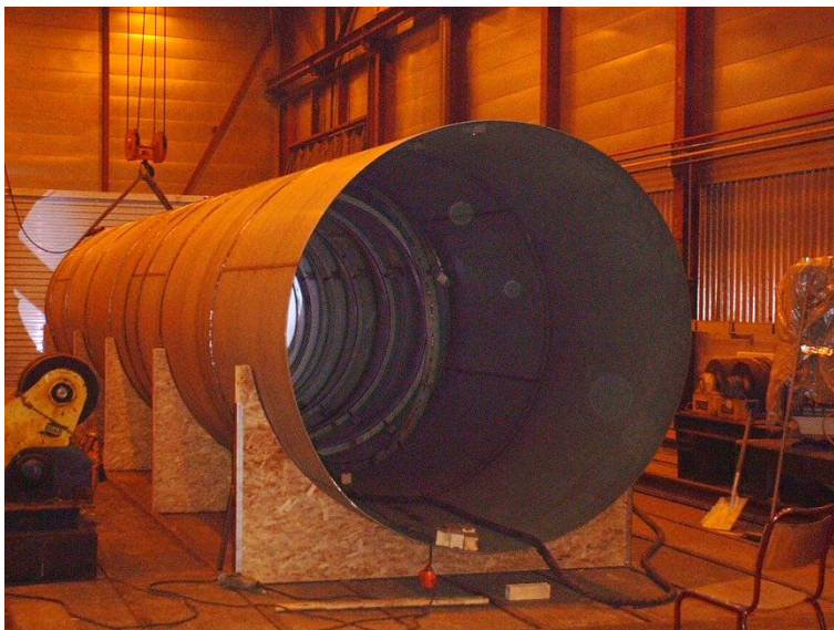
Lined duct for exhaust – fabrication in workshop
