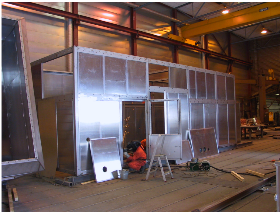
Assembly of panel noise hood in our workshop
