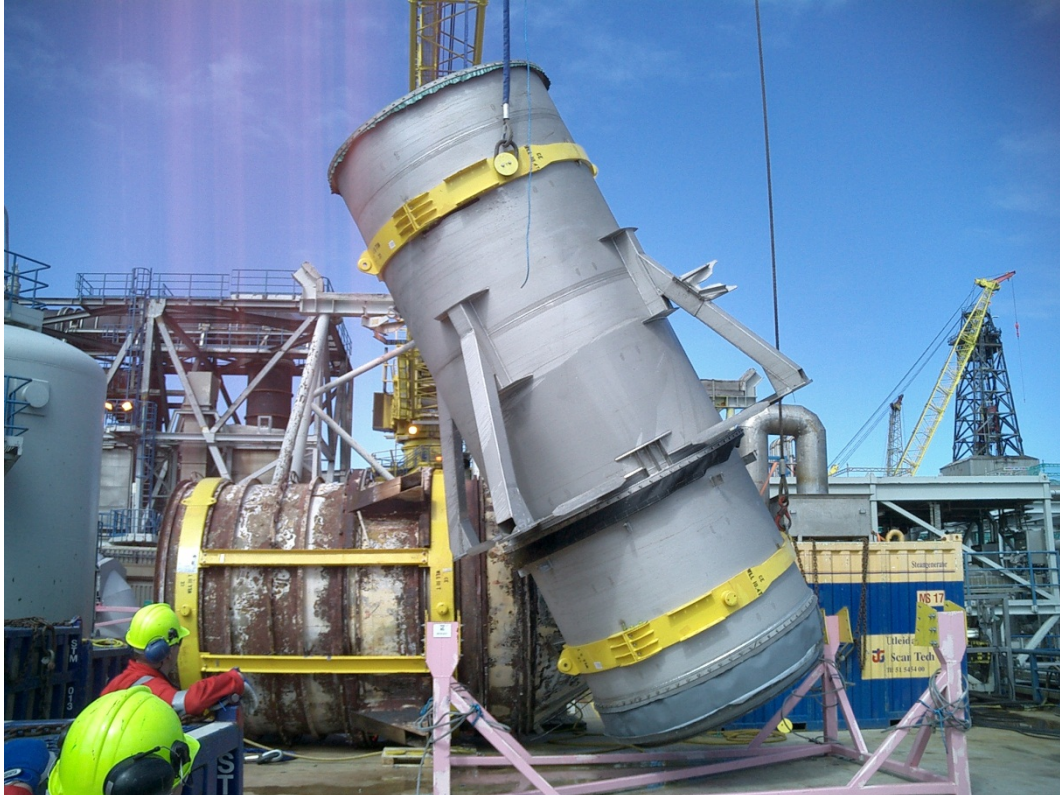
Oseberg A – HTB – transport frame and lifting tool
