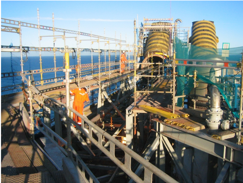
Oseberg HTA exhaust system – dismantling old system
