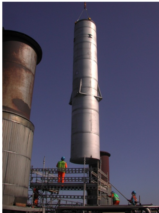
BP Valhall – mounting of the new exhaust stack into the module
