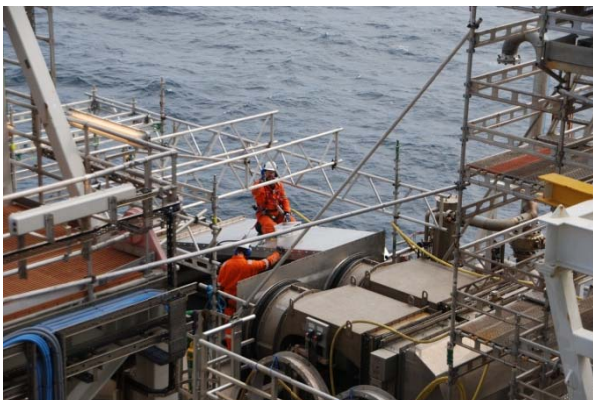
Visund – modification on the ventilation and anti-ice system
